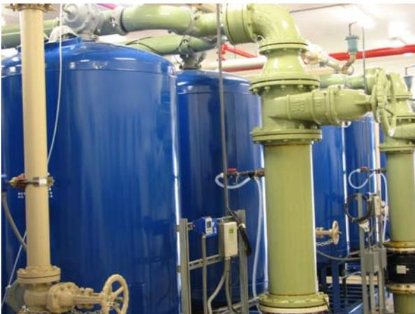
The filtration method at Plant No. 2 utilizes chlorine, which oxidizes the iron allowing it to be filtered, and special sand that the iron bonds to as the water passes through the filter. The finished water from the filters is chlorinated, fluoridated and blended in the 100,000-gallon mixing tank with finished water from Plant No. 1.
